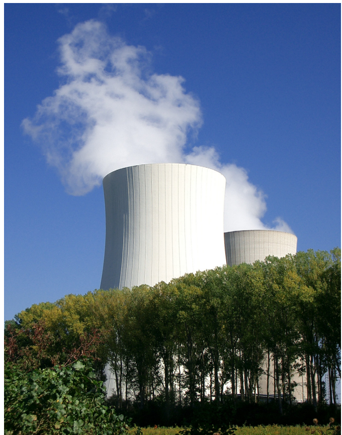
Fig. 2: Typical application: Power plants
